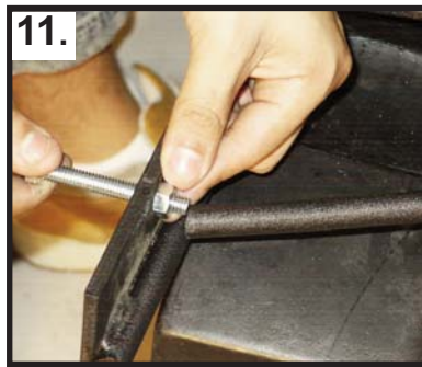
Put the 2 1/2" hex bolts thru the axle and start threading on 4 nuts.
